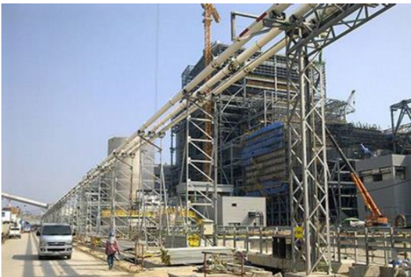
Figure 2: Example of an overhead GIL installation (left) and typical pipe bridge (right).
