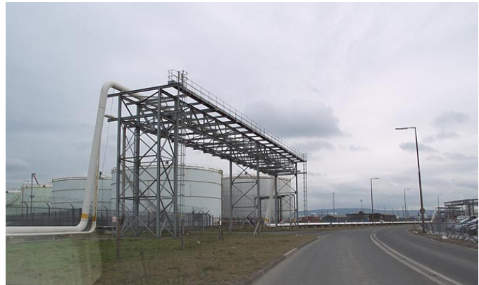
Figure 2: Example of an overhead GIL installation (left) and typical pipe bridge (right).
